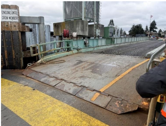
Anacortes Bridge Apron
